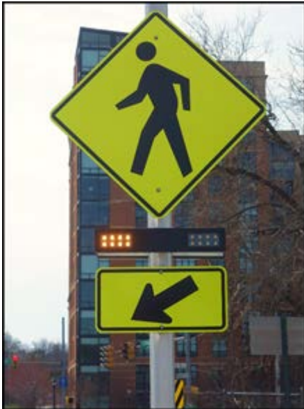
Exhibit 3.4 – Rectangular Rapid Flashing Beacon
