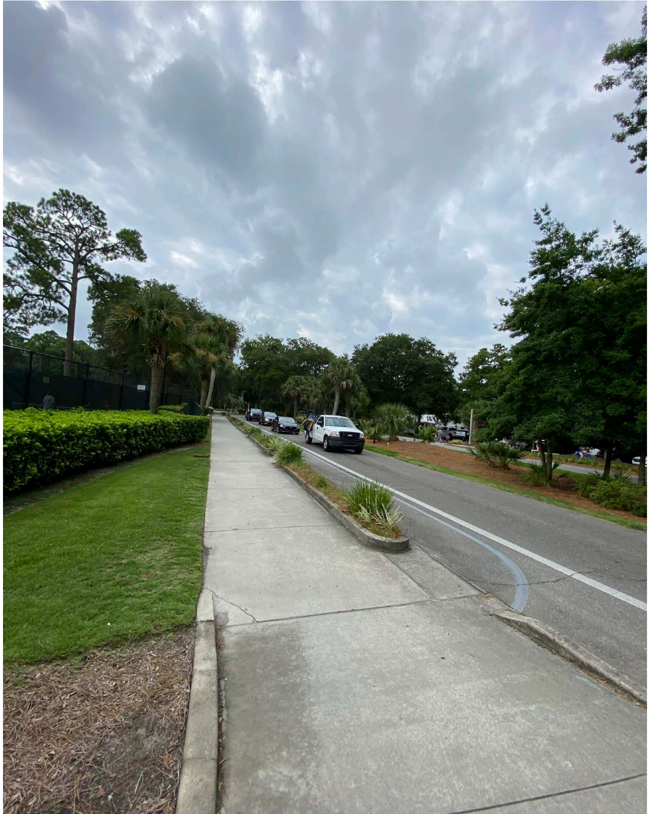
Exhibit 3.11 – Queens Folly Road Observation Photo #19
