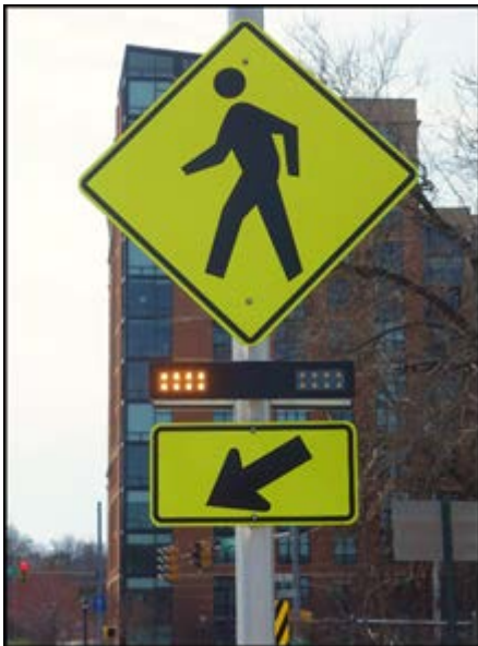
Exhibit 3.4 – Rectangular Rapid Flashing Beacon
